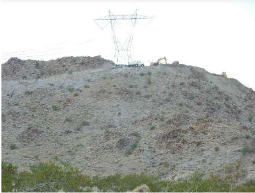
**Figure 3.** Grading/site clearing activities at Tower 2416.
